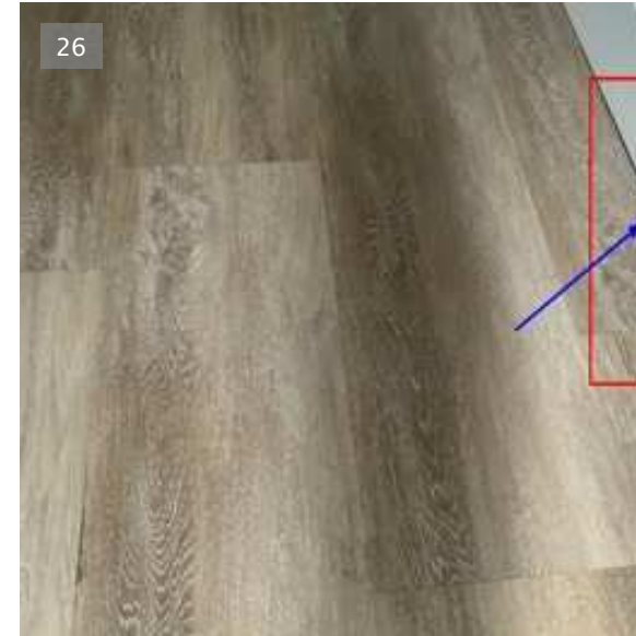
Edging quadrant or sealant recommended between floor and skirting 18/01/2021 10:00 (GMT) at 52.131084589851234°, -0.012110049585854777°
